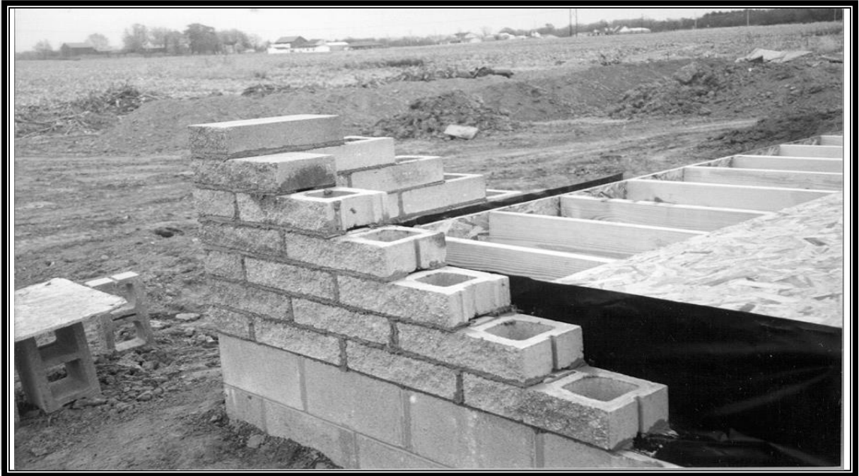
FIGURE 1.6 House Construction Using Concrete Masonry
