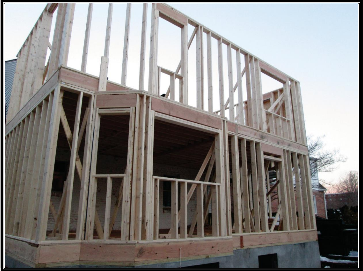
Modern Platform-Framed House Under Construction
