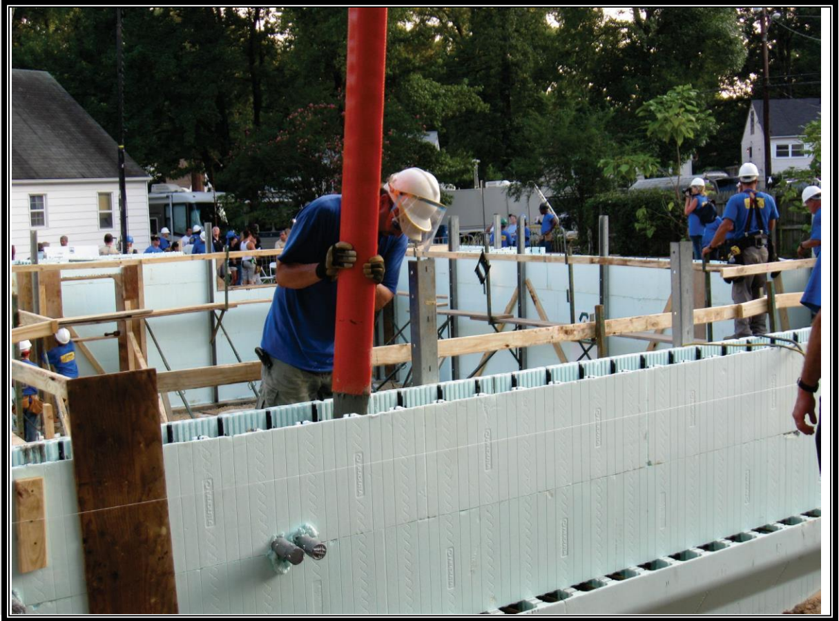
House Construction Using Insulating Concrete Forms
