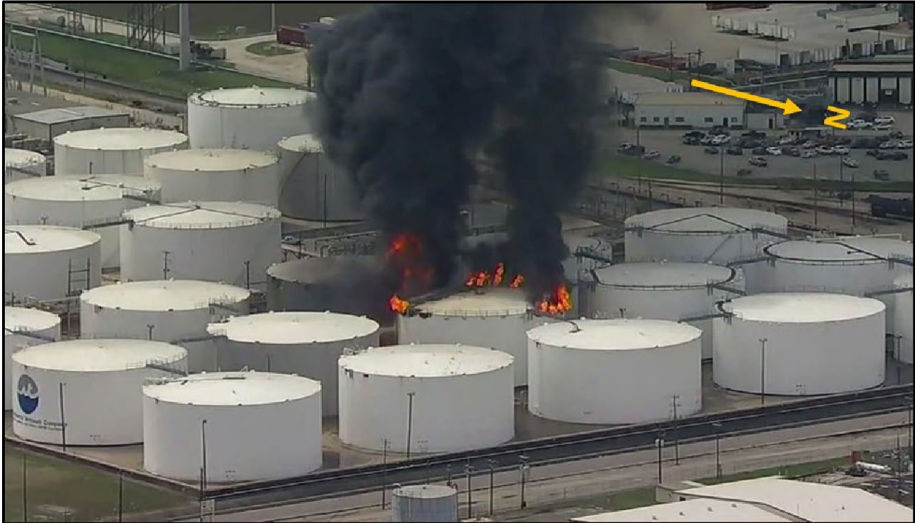
Figure 12. ITC fire involving Tank 80-8 on the morning of March 17, 2019. (Credit: ABC13 Houston, annotations by CSB)
