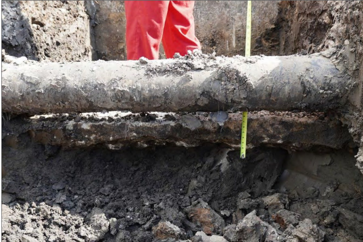
Photo 23: Containment wall footing and underside of footing
