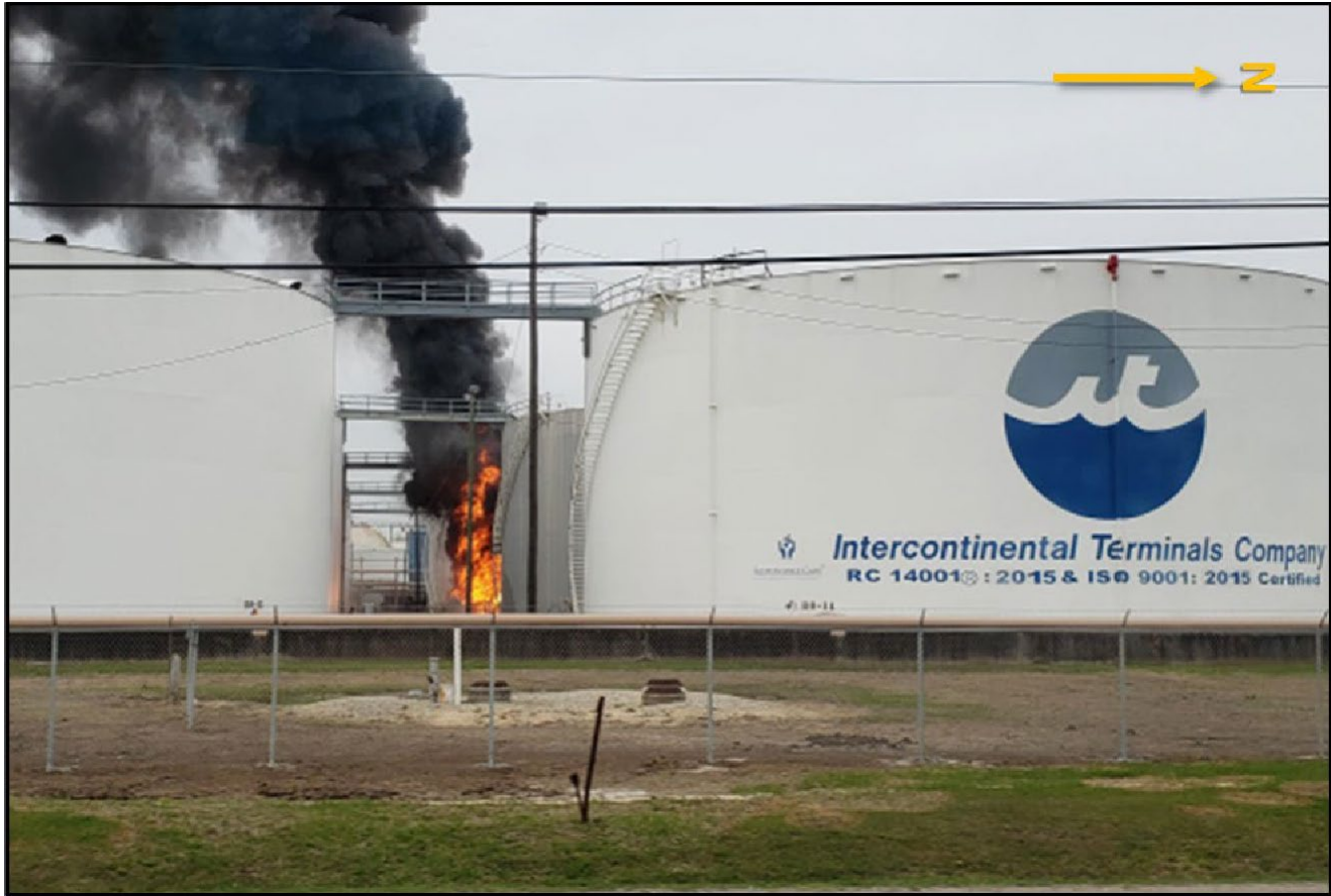
Figure 11. Initial ITC tank fire that ignited at Tank 80-8 on March 17, 2019. (Credit: HCFMO, annotations by CSB)
