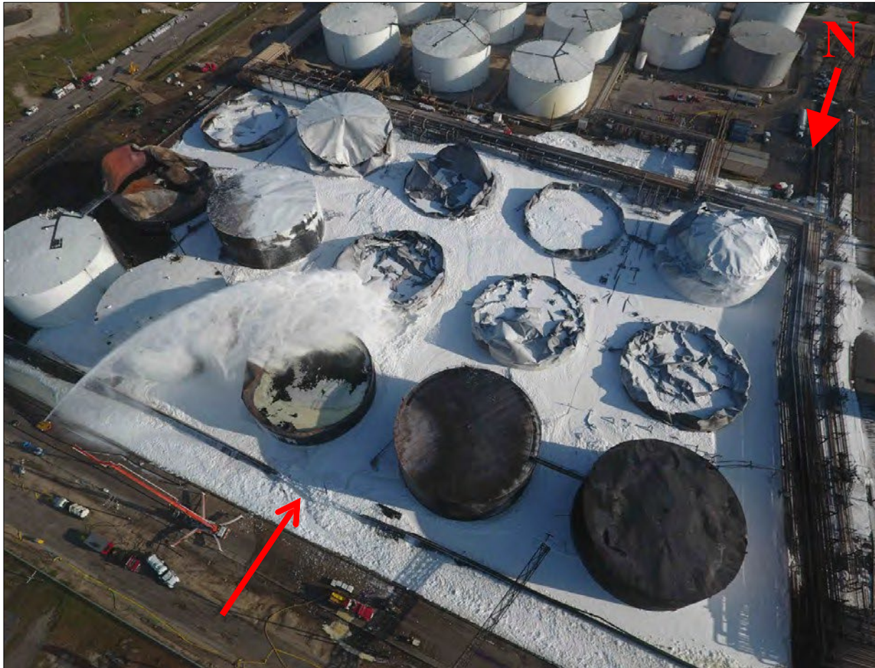
Photo 4: Containment wall failure (red arrow) during fire suppression efforts 12
