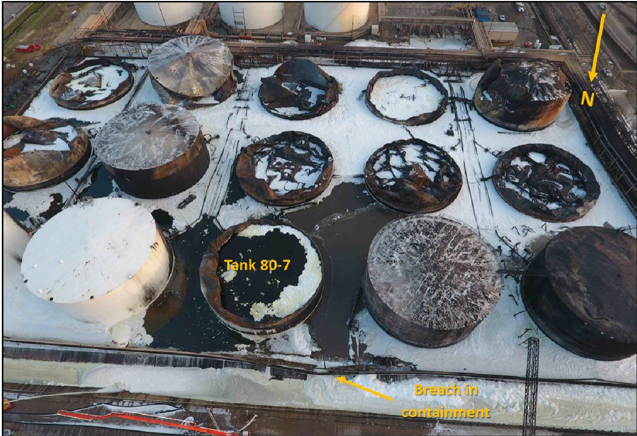
Figure 16. Overhead view of the First & Second 80's tank farm containment wall failure that allowed materials to enter the surrounding waterways on Friday, March 22, 2019. (Credit: ITC, annotations by CSB)
