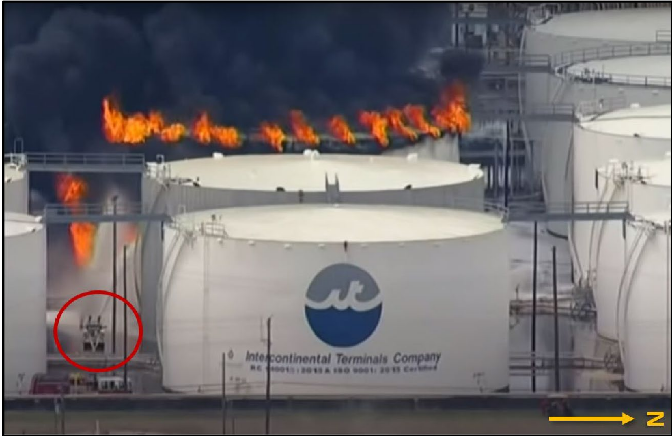
Figure 13. The quick attack truck (circled in red) staged between Tanks 80-11 and 80-12 on March 17, 2019. (Credit: Associated Press, annotations by CSB.)
