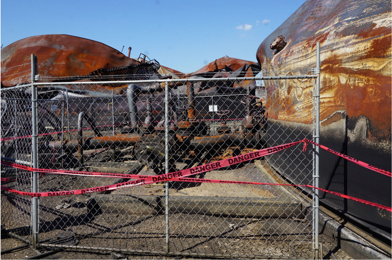
Figure 30. Small concrete containment area around the Tank 80-8 circulation pump. (Credit: CSB)
